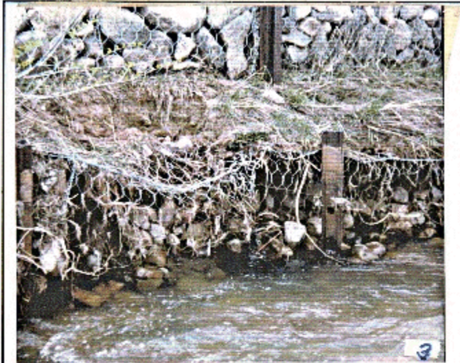
Figure 40. Damaged gabions
