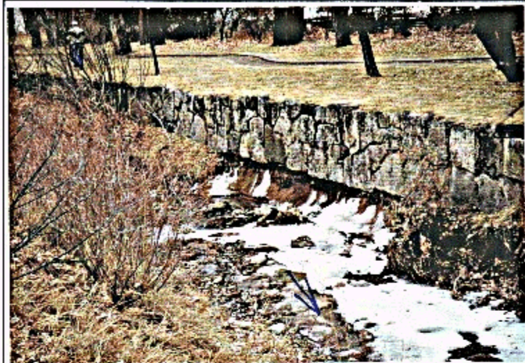
Figure 5. Suspended rock wall
