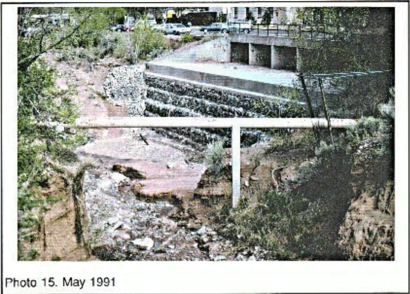
Sewer Line Crossing 11
