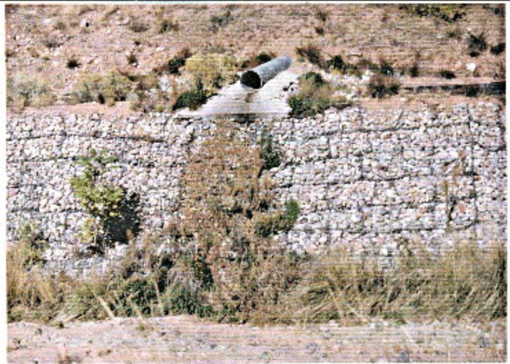
Figure 32. Stormwater rundown
