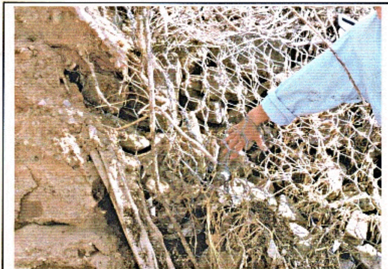
Figure 41. Lost rockfill
