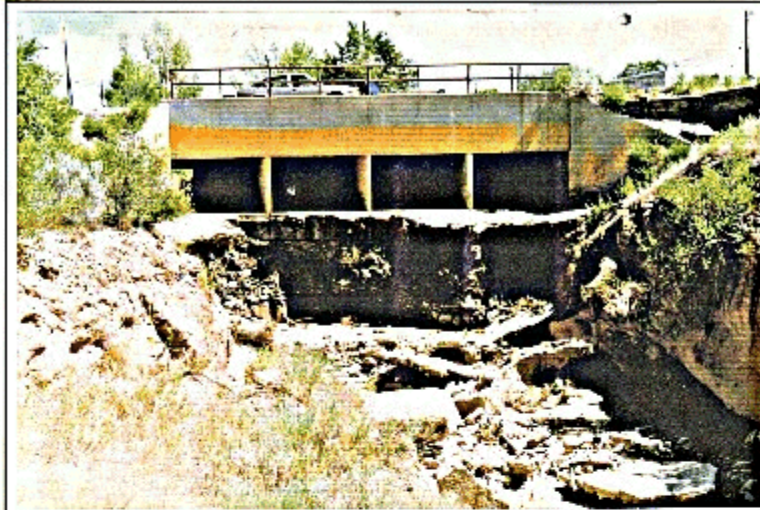
Figure 17. One way to halt a headcut
