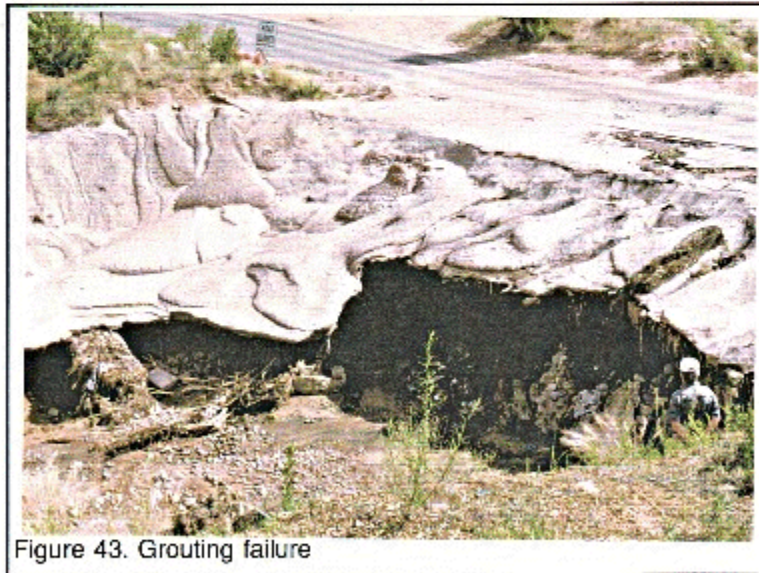
Figure 42. Grouting failure
