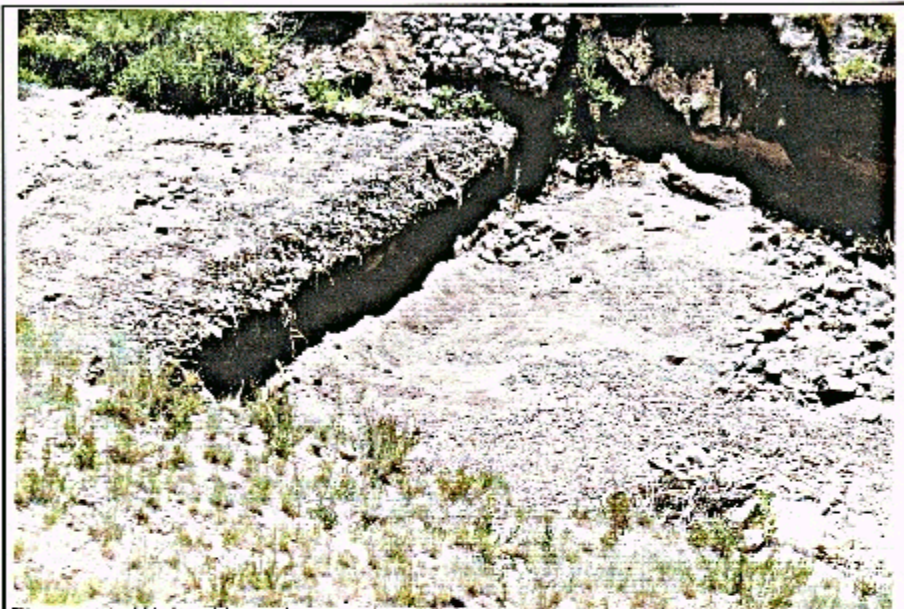
Figure 10. Weir with end protection
