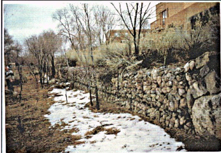
Figure 36. 25-year gabions in "as built" condition
