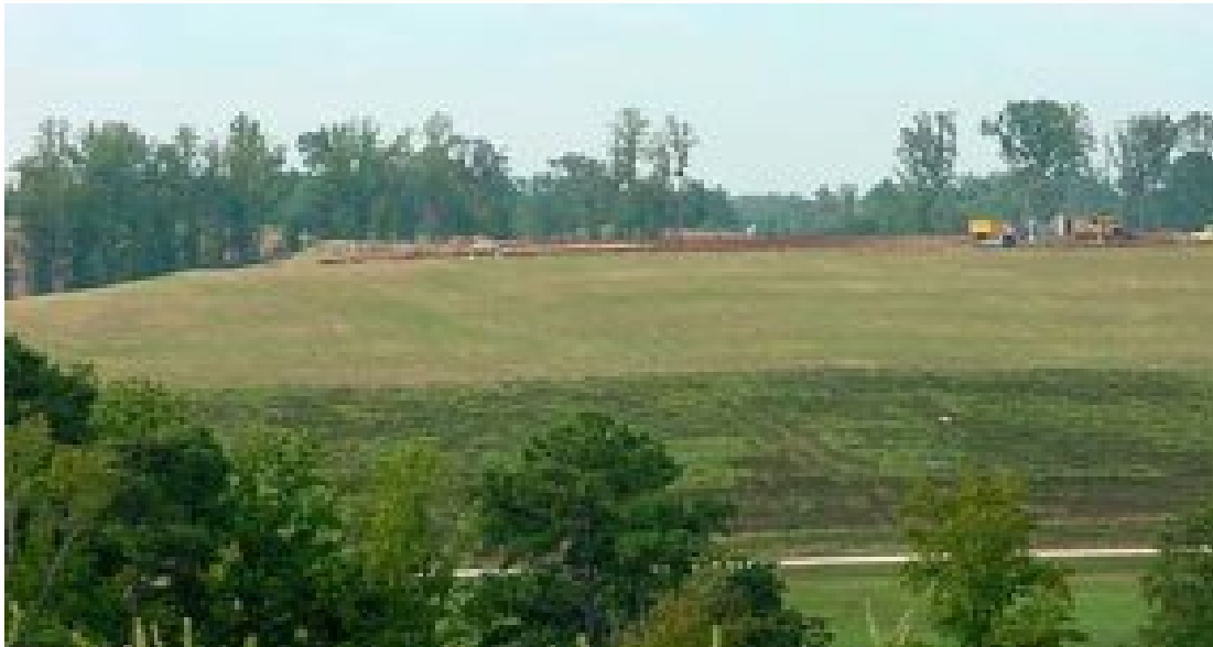
Figure 31: Grass and other plants cover at the completed landfill
