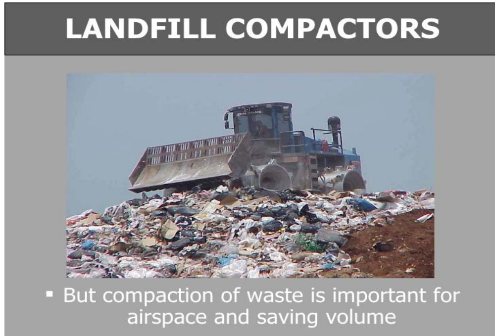
Figure 7: Landfill Compactor being used in working face
