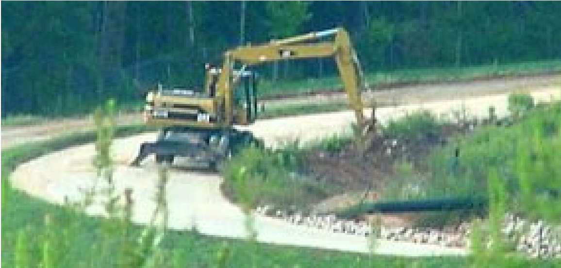
Figure 16: Drainage ditches run along the base of a landfill. Controls both run-on and run-off
