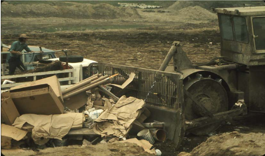
Figure 6: Steel-wheeled compactor spreading waste in a working face
