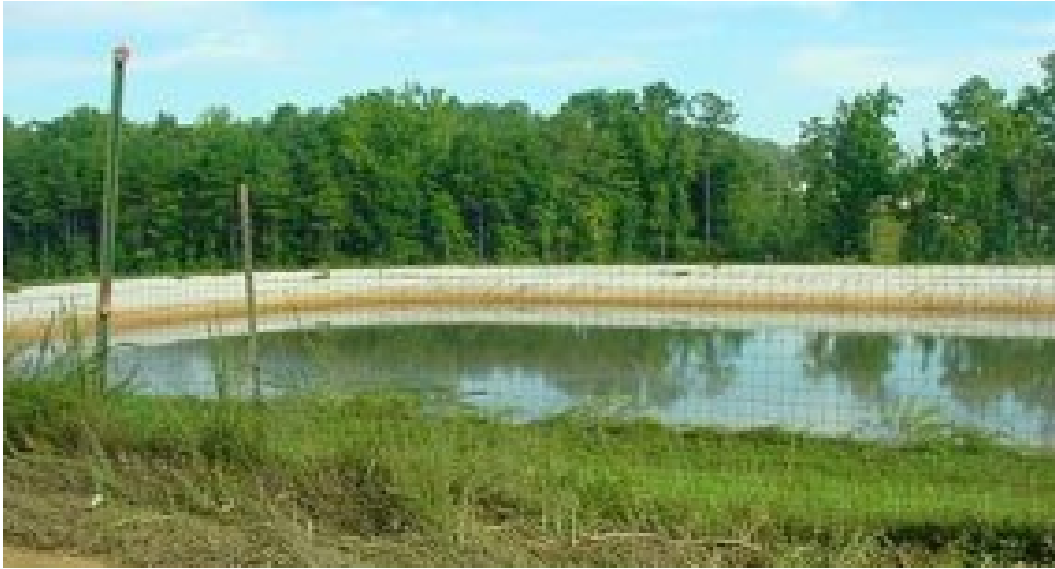
Figure 12: A leachate collection pond is designed to catch the contaminants that can get into water that goes through the trash in a landfill
