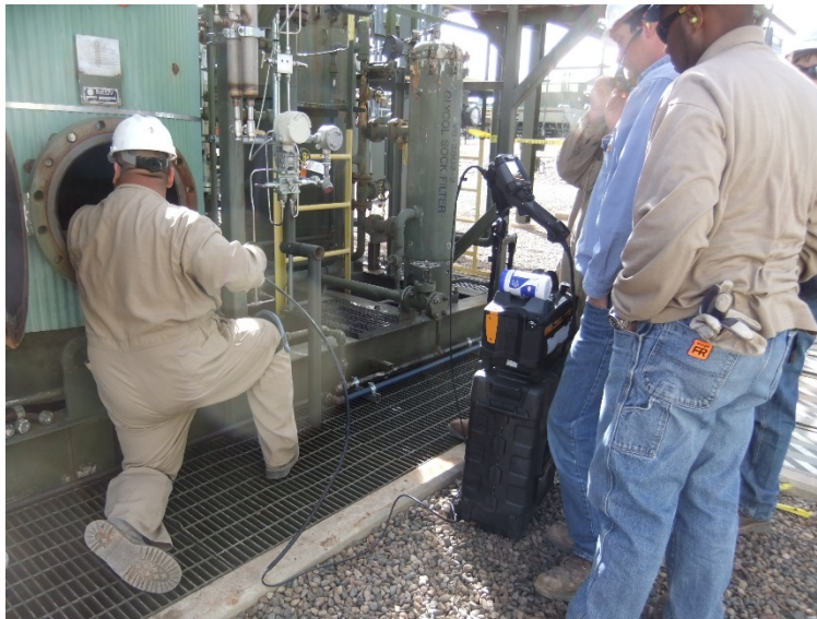
Figure 25 Internal inspection of vessel using an articulating borescope
