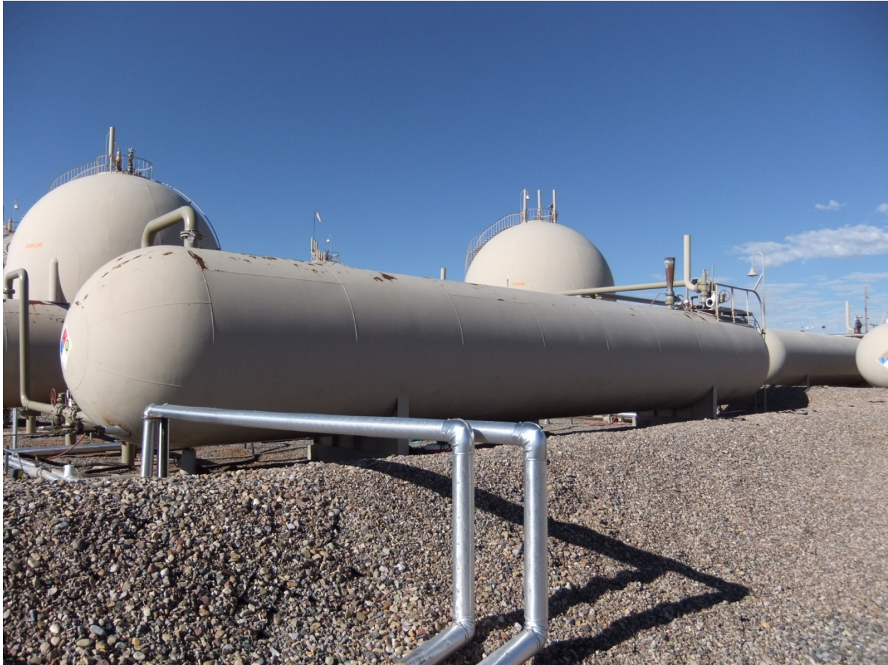
Figure 22 View of liquids storage bullet tank at a major oil and gas producer's natural gas processing facility. Vessel built in 1955 by Riley Beard and still in service in 2011.
