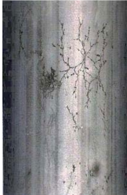
Figure 9 Close-up view of tight web appearing SSC cracks on Type 316L SS tubes in steam service [8].
