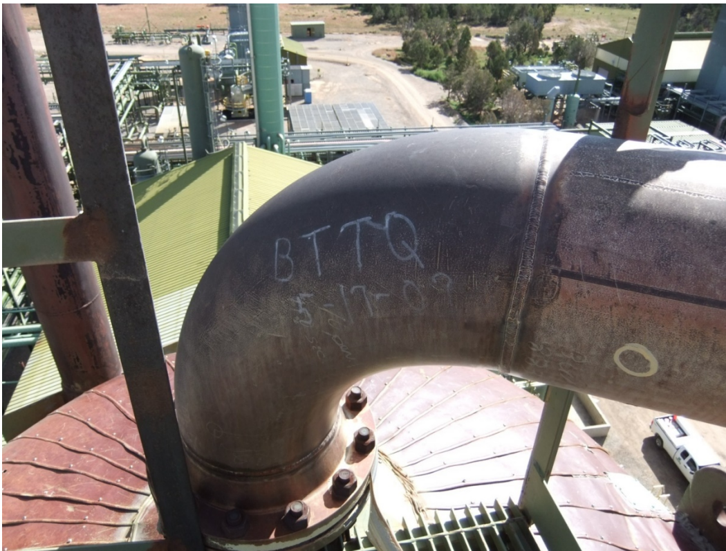
Figure 18 View of outlet piping at top of amine contactor tower at a major oil and gas company natural gas treating facility.
