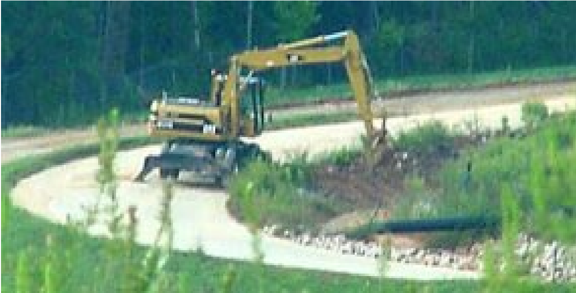
Figure 41: Drainage ditches run along the base of a landfill. The black pipe carries landfill gas to a pumping station. Controls both run-on and run-off
