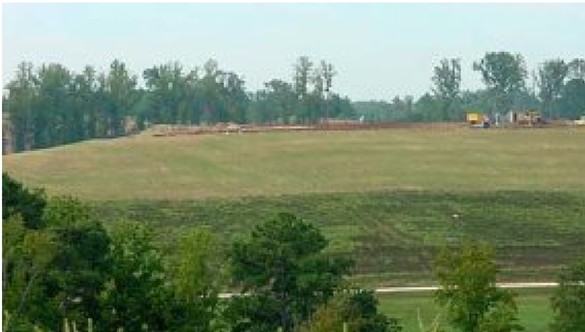
Figure 42: Grass and other plants cover at the completed municipal solid waste landfill
