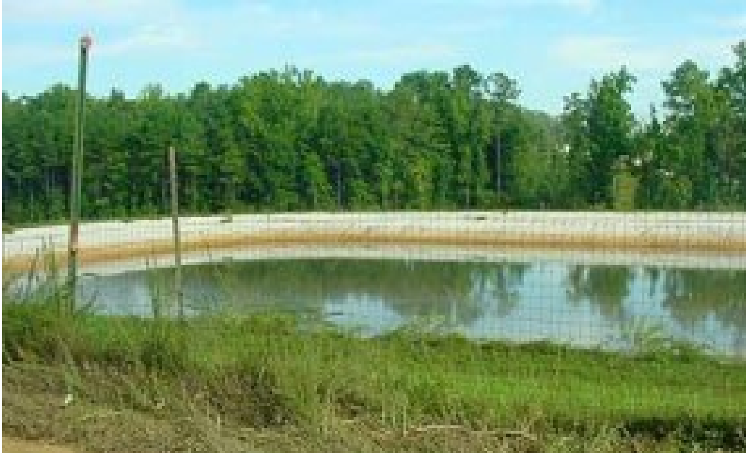
Figure 32: A leachate collection pond is designed to catch the contaminants that can get into water that goes through the trash in a landfill
