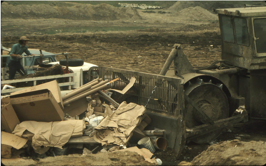
Figure 7: A Steel-wheeled compactor spreading waste in a working face
