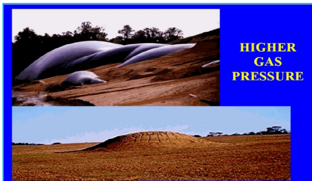
Figure 39: Effect of landfill gas pressure on final cover
