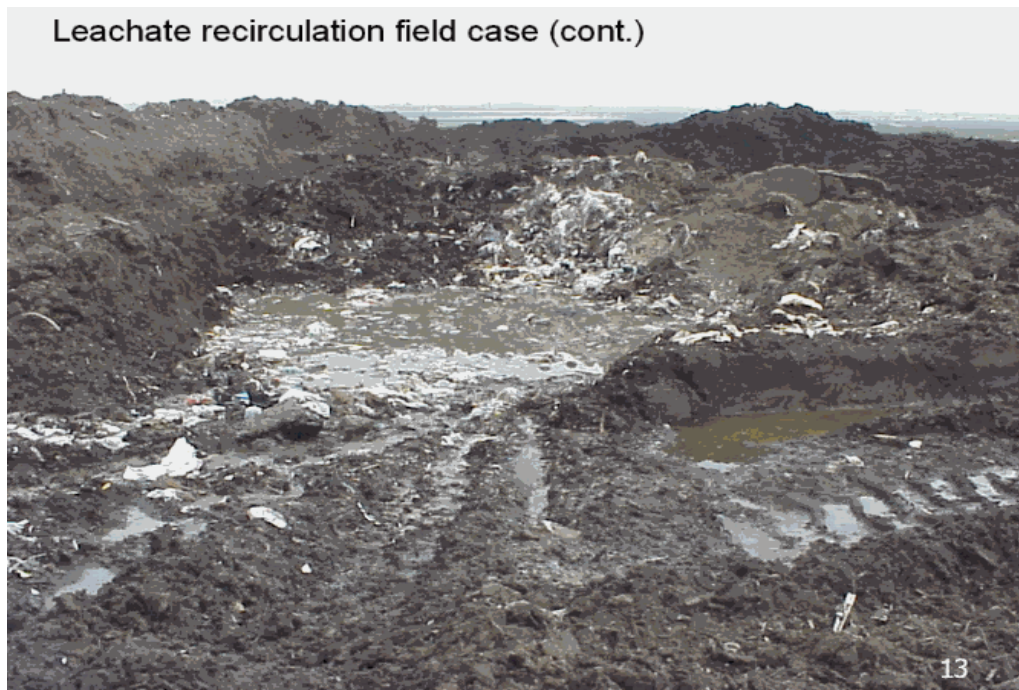
Figure 18: Ponding Used in Landfill
