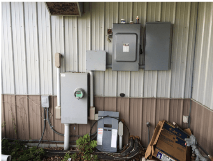
Figure 136 - Example Supply-Side Interconnection
