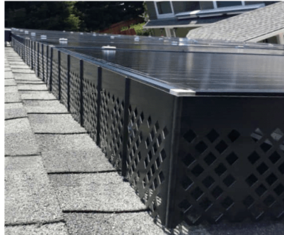
Figure 77 - Snow Guard and Array Skirt
