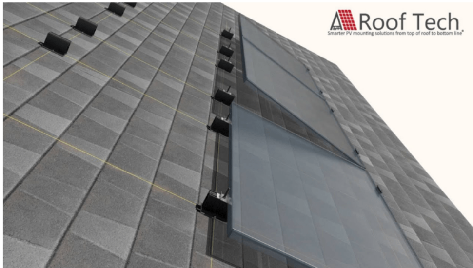
Figure 46 - Rail-less Racking Example
