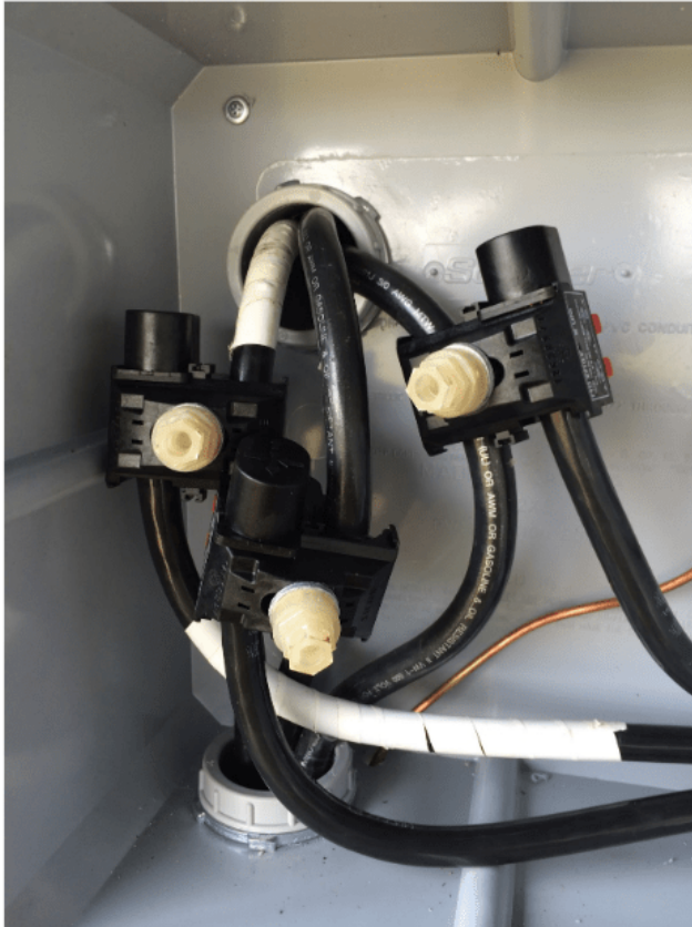
Figure 137 - Insulated Tap Connectors
