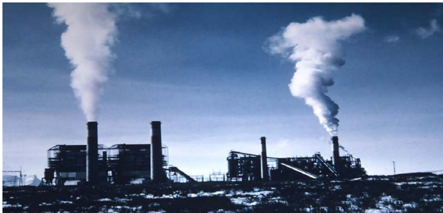
Figure 32: Electrostatic precipitators (ESPs) in service in a power plant
