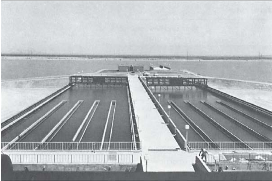
Rectangular settling tank with longitudinal weirs 1
