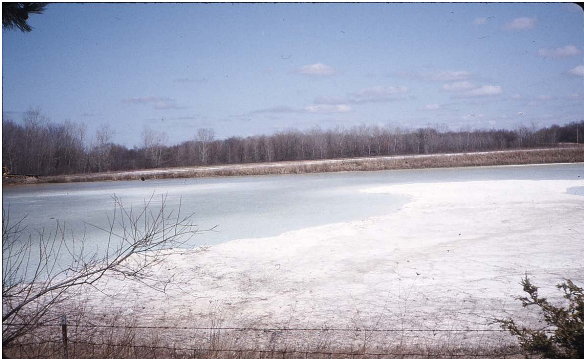
Softening sludge lagoon. Winter view shows ice (light blue) where supernatant water is standing.
