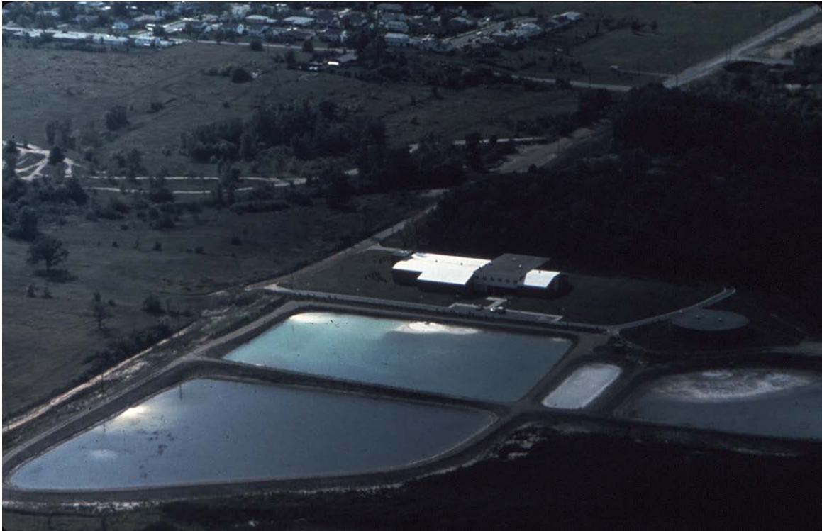
Overview of water treatment plant showing sludge lagoons and building housing treatment facilities.
